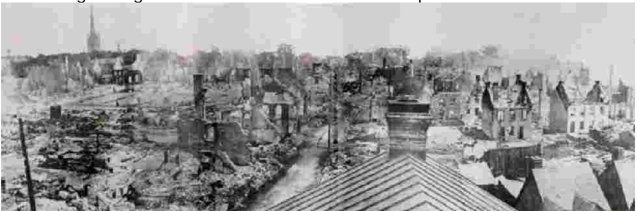
Crumbling shells of homes and businesses are all that remains after a fire razed much of Trois-Rivières in 1908.
